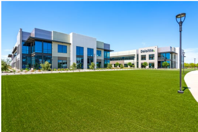
Deloitte's buildings at Gilbert's Rivulon campus. (Photo: Courtesy of Nationwide Realty Investors)
