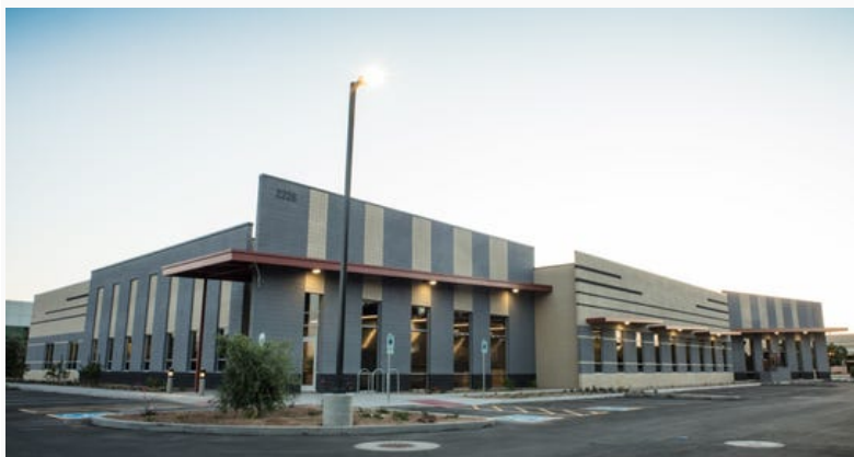
Moog's new building at 2228 West Guadalupe Road in Gilbert. (Photo: Courtesy of Willmeng Construction)
